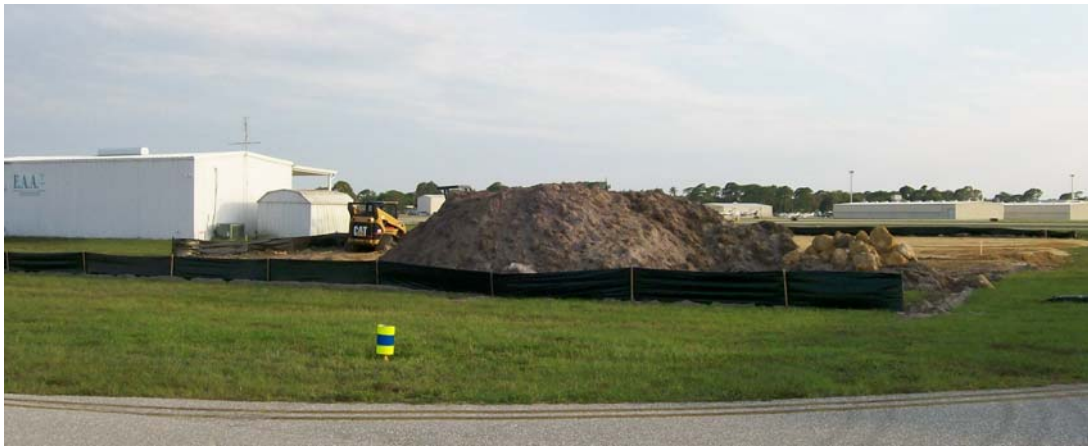
Our new neighbors DEAN STEEL starts construction
